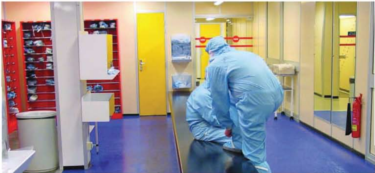
Dycem CleanZone Blue covers the whole changing area at electronics giant Philips.
